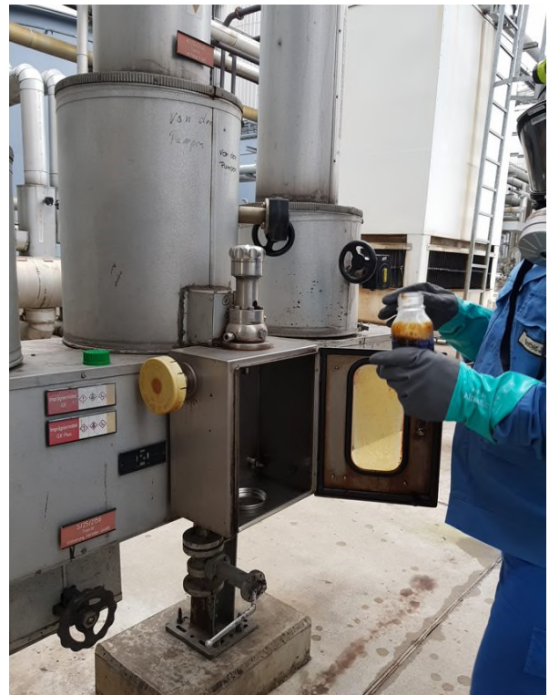
Figure 15-12 #B Removal of sampling vessel - 2
