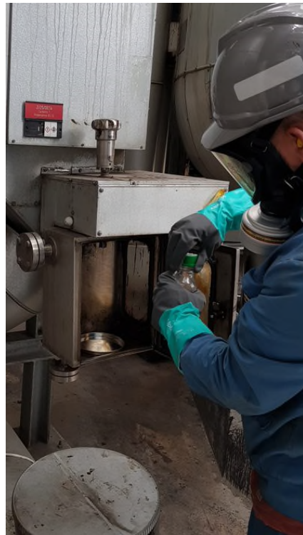
Figure 15-8 #A Closing sampling vessel
