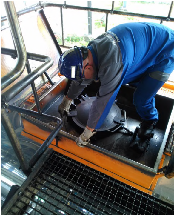
Figure 16-1 Worker opening manhole - 1
