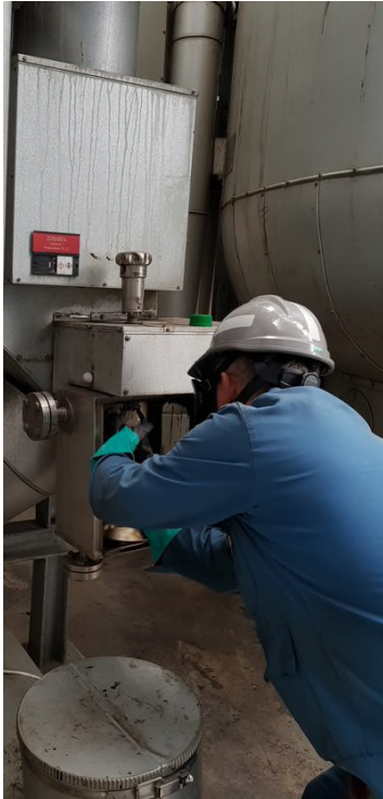
Figure 15-5 #A Installation of sampling vessel
