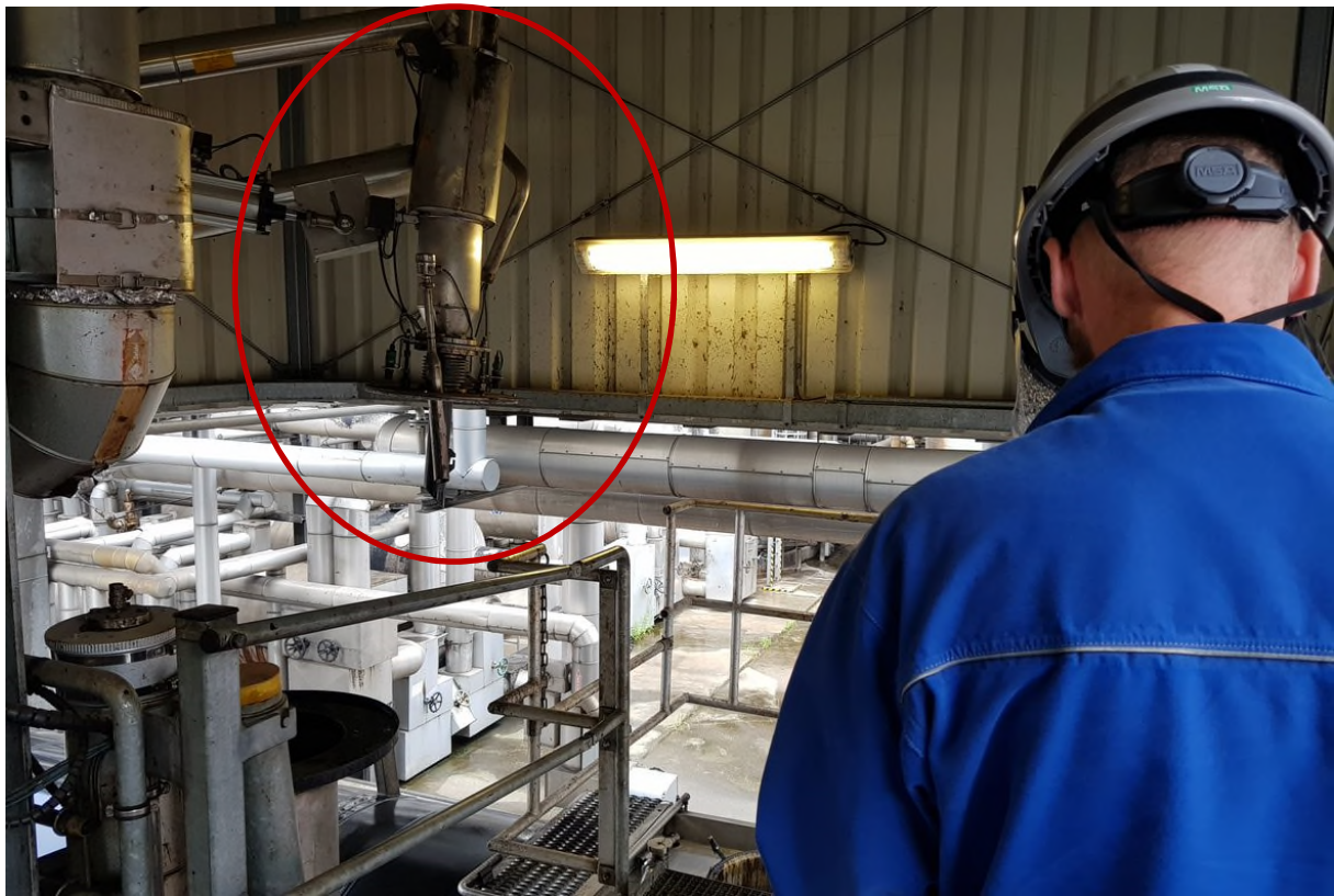
Figure 16-5 Worker starting automated movement of loading arm - 1
