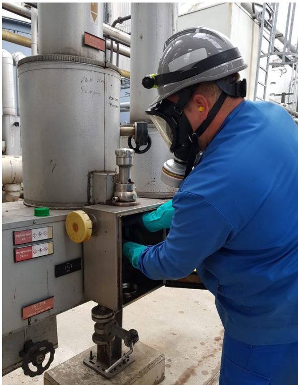
Figure 15-11 #B Removal of sampling vessel - 1
