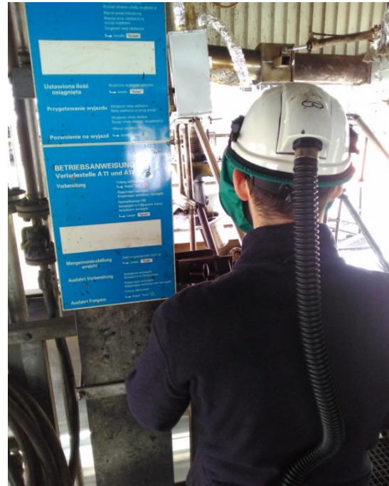
Figure 16-9 Worker operating loading arm after loading completed
