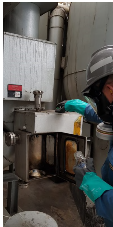
Figure 15-4 Opening closed sampling point #A (no exhaust ventilation)
