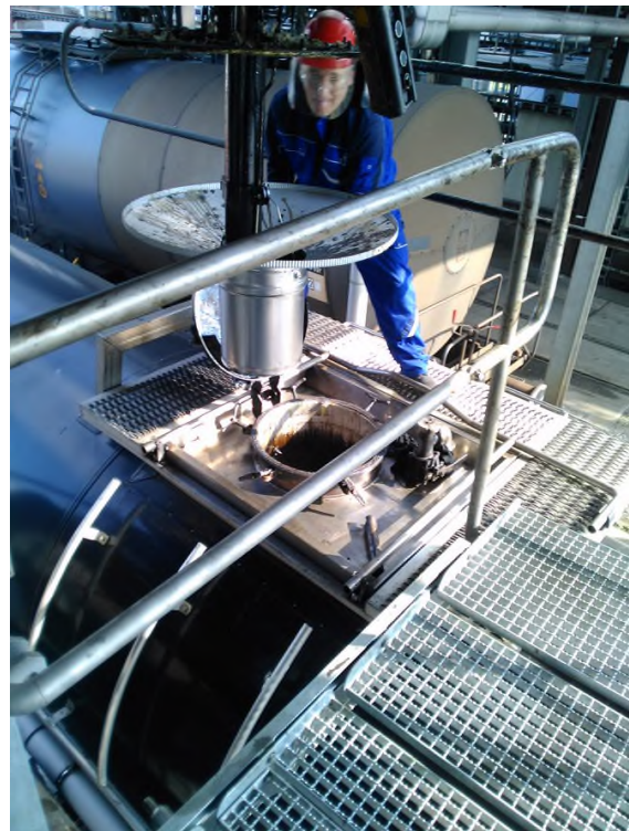
Figure 16-4 Worker removing drainer before loading
