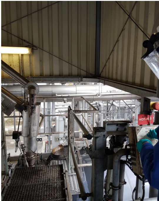
Figure 16-8 Loading arm final placement
