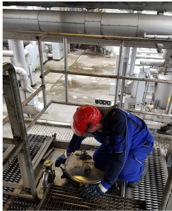
Figure 16-2 Worker opening manhole - 2
