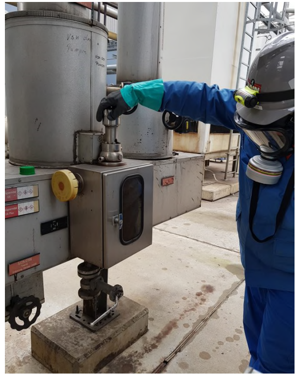
Figure 15-10 #B opening substance flow and visual inspection of filling
