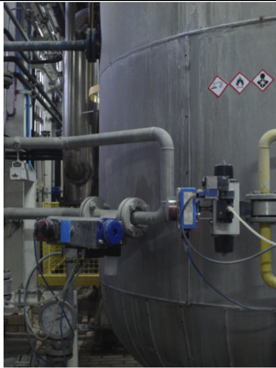
Figure 6 Closed sampling loop
