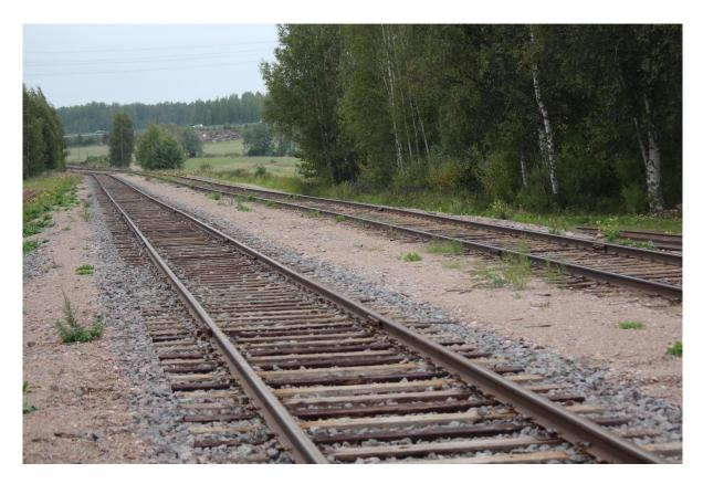
Figure B - 12: Reused wooden sleepers, Lapinjärvi, Finland, August 2021 (source: FTI Finland)
