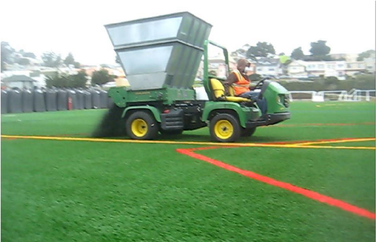
Figure A 9: Semi-mechanised application of infill
