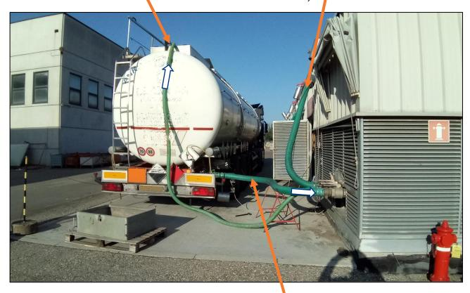
Unloading pipework to transfer enamel from road tanker to enamel storage tank
