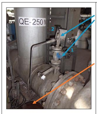
Double block valve (1: gate valve, 2: needle valve)
