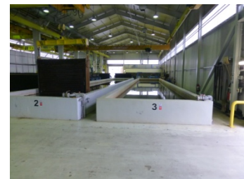
Storage Pits filled with water
