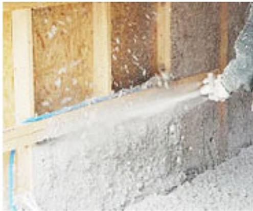
*Figure 5: Illustration of cellulose insulation flocking (NrGaia website, 2013)*
